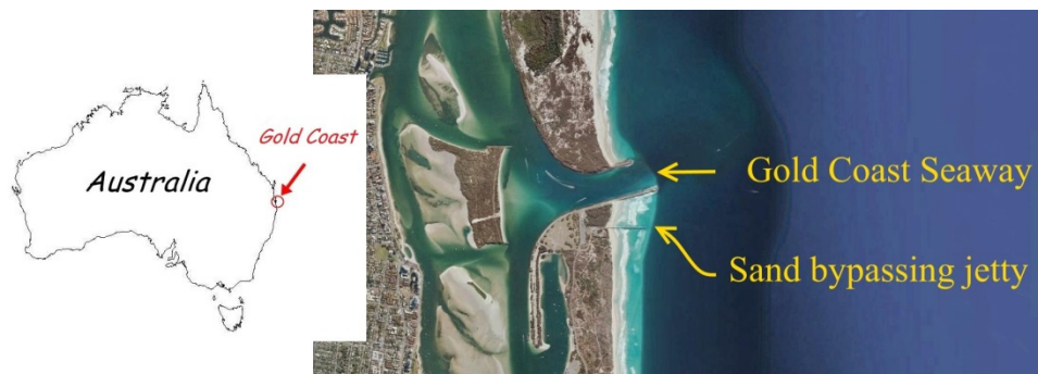
Figure 1. Gold Coast Seaway and the Sand bypassing system location
