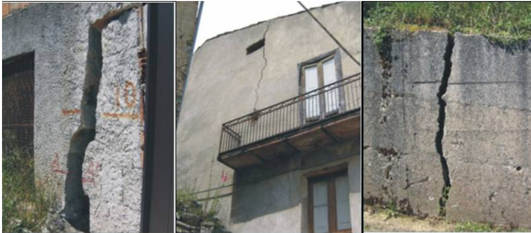
Figure 3. Fractures on buildings and constructions in San Martino di Finita.
