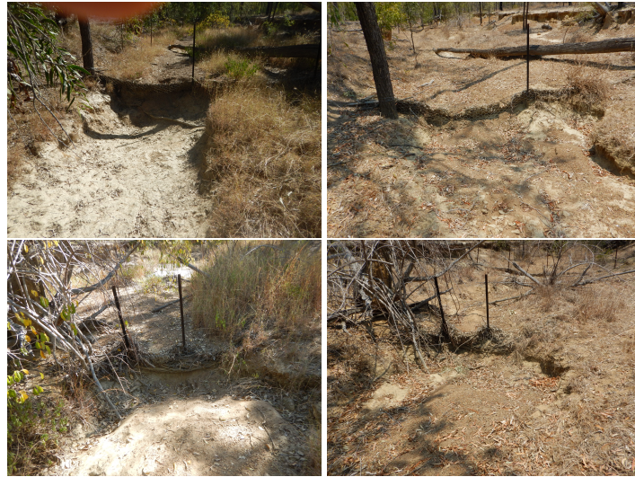
Figure 1. Photos at two porous check dam sites in the Fitzroy River Basin taken approximately 18 months apart. In these cases, the earlier photos (left) show significant scouring below the PCDs, which is later covered by sediment and leaf-litter providing a protective barrier against further erosion. Photos © K. Roots.
